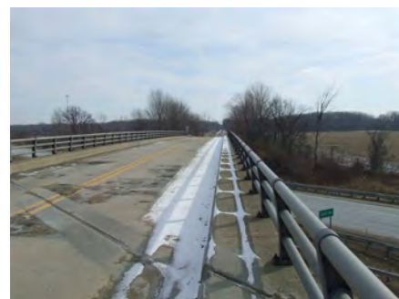
25 East at I-94 Bridge
