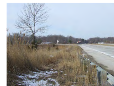
33 US-12 @ railroad looking west
