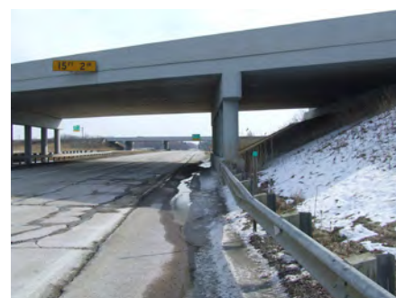
34 US-12 @ I-94 looking east
